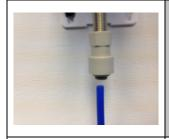
Screw the quick connect tap adaptor' hand tight' to the stud of the tap. Nip up the adaptor with a spanner (do not overtighten) Connect a length of blue tubing between the quick connect tap adaptor and the outlet of the module (O).
