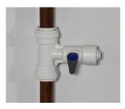
Identify a suitable length of 15mm mains cold water pipe work that is straight, clean and free from paint. Turn off the supply, drain down the pipe and remove sufficient pipe to allow for the pushfit tee to be fitted. The cuts to the tubing should be square and free from burrs. Ensure that the lever valve to the ½" branch is turned off before the water supply is turned back on.
