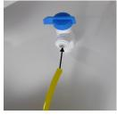
Connect a length of yellow tubing between the storage tank valve (11) and the post filter inlet tee.
